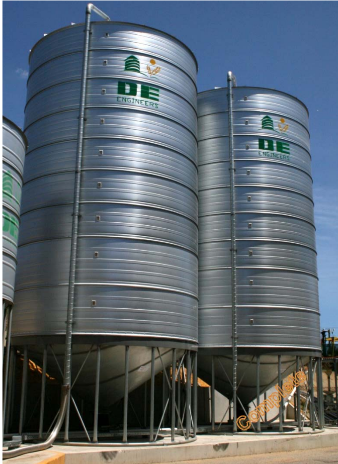
2x100 tonne malt silos
